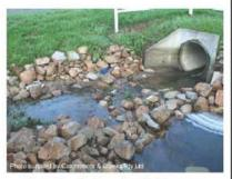
Photo 1 - Rock stabilised pipe outlet
